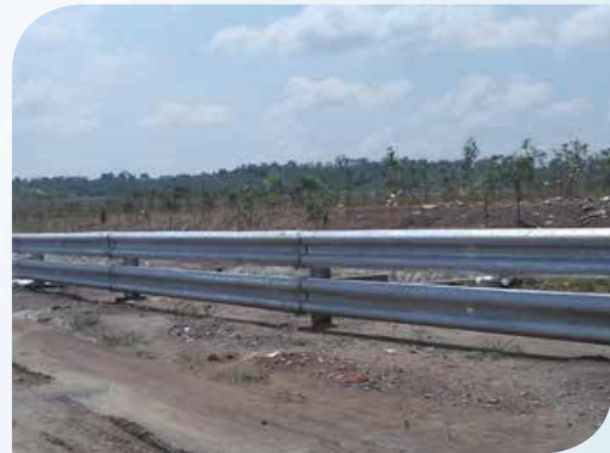
FLEX BEAM GUARDRAIL
